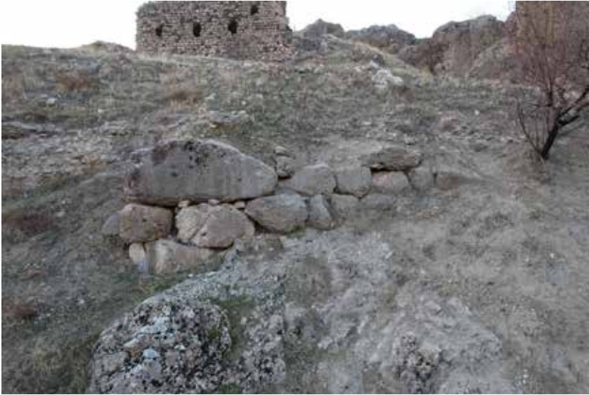
Figure 7: Remains of the terrace wall that separates the Upper Citadel from the Lower Citadel.
