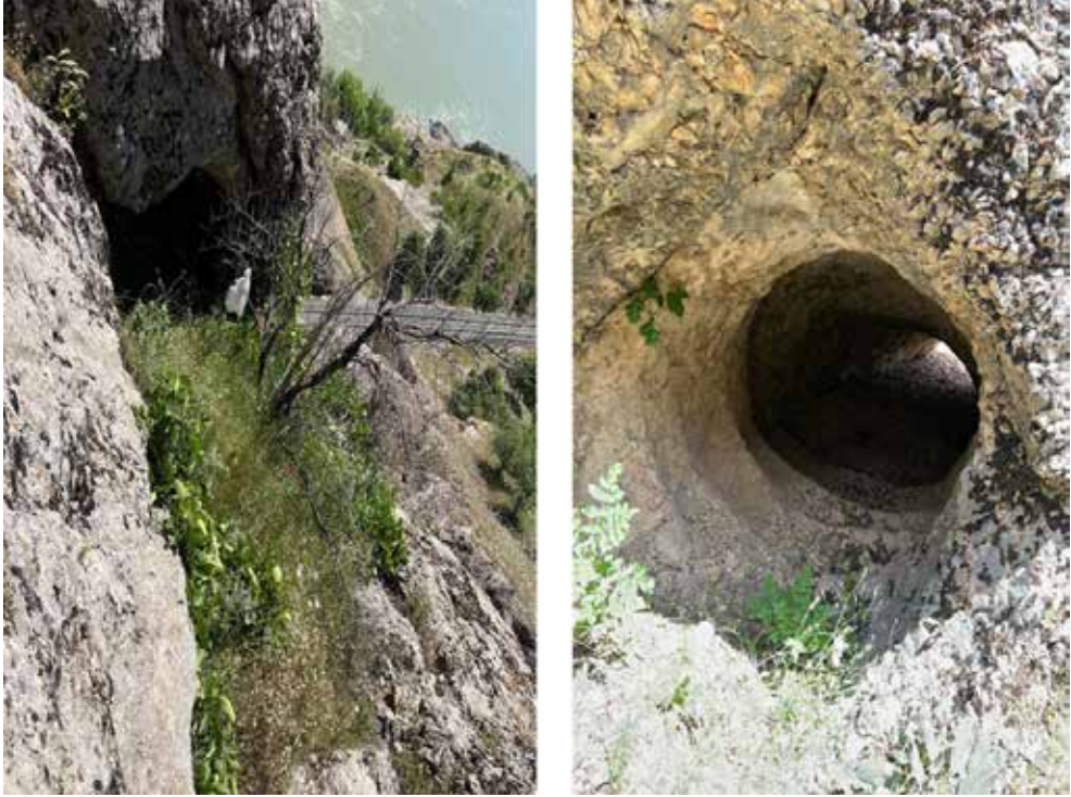
Figure 23: Entrance to Stepped Rock-cut Tunnel C (left), view from inside the tunnel (right).
