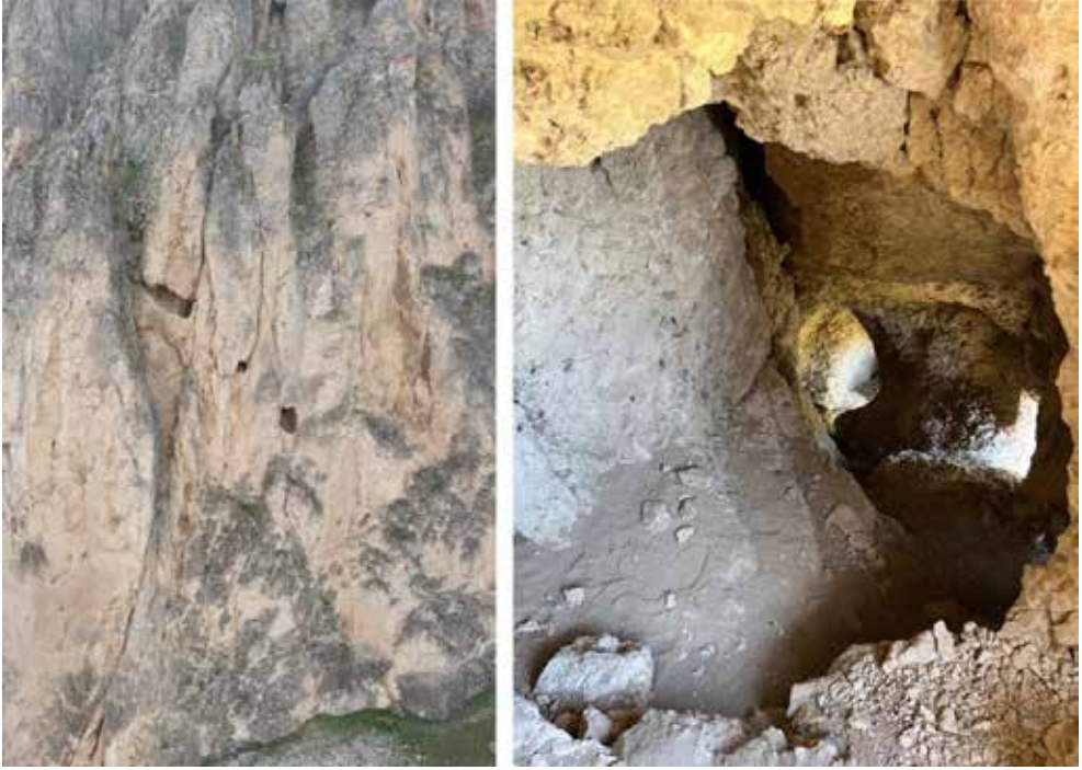
Figure 24: Exterior view of Stepped Rock-cut Tunnel D (left) and interior of the tunnel (right).
