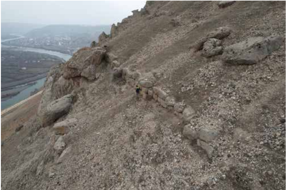
Figure 10: Lower Citadel fortifications, view from the northeast.
