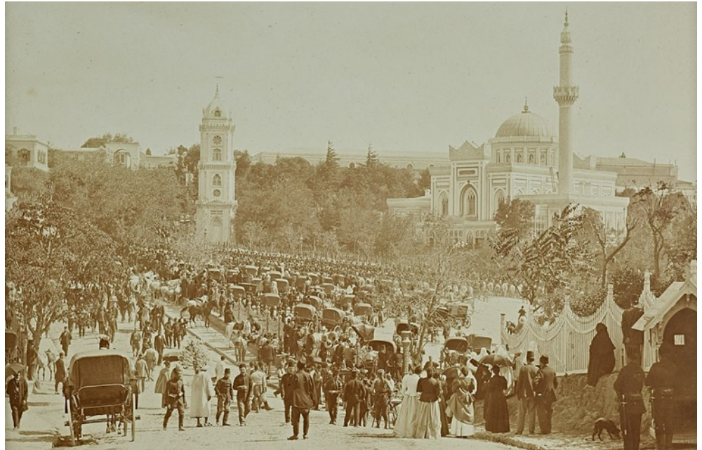
Figure 14. Hamidiye Mosque and the clock tower (IU, YPA)
