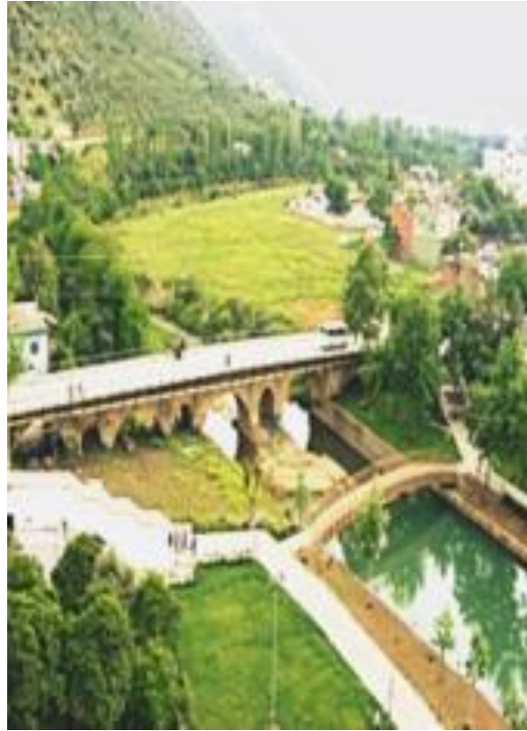
Figure 3. The Upstream Façade of Kozan Bridge (Photo: İ. Göçmen)
