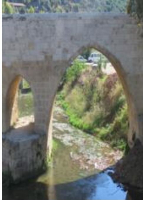
Figure 8. Detail of the Third Arch of the Bridge (Photo: İ. Göçmen).
