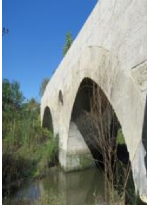
Figure 11. Second Arch of the Bridge (Photo: İ. Göçmen)
