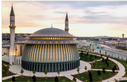
Figure 30 Ali Kuşçu Mosque at İstanbul Airport ( https://www.istairport.com/hizmetler/deneyim/ortak-ihitiyaclar/ibadethaneler/ )
