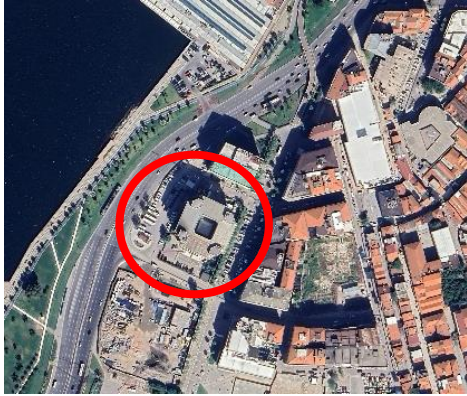
Figure 5. Central Bank google maps image, 2023 [26]
