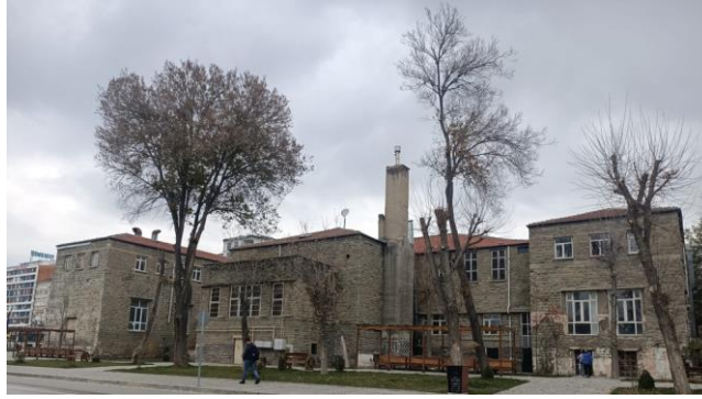
Figure 22. The current southern facade of the building [19]
