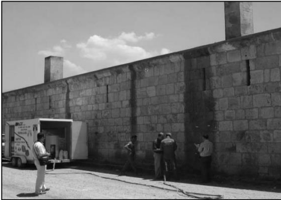
Figure 11. Process of Determining the Surface to be Micro Sandblasted [37]
