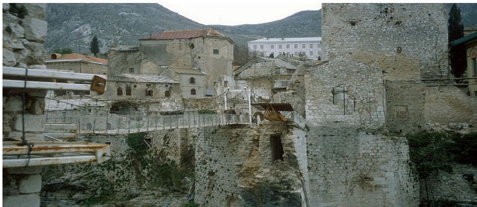
Figure 3. Temporary Bridge After Destruction
