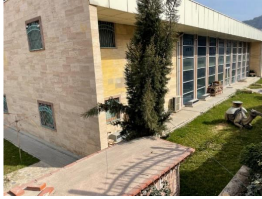
Figure 4. Tokat City Museum South-West Facade (S. Seyfi, 2024).
