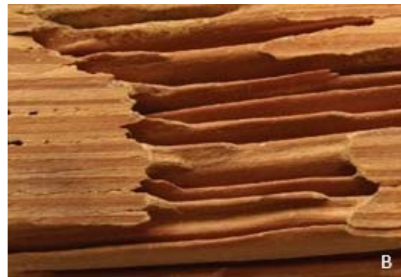
Figure 10. Termite damage on pine (Arango et al., 2021).
