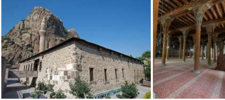
Figure 3. Figure 4. Afyonkarahisar Ulu Mosque general view and interior (Kültür Envanteri, 2024).
