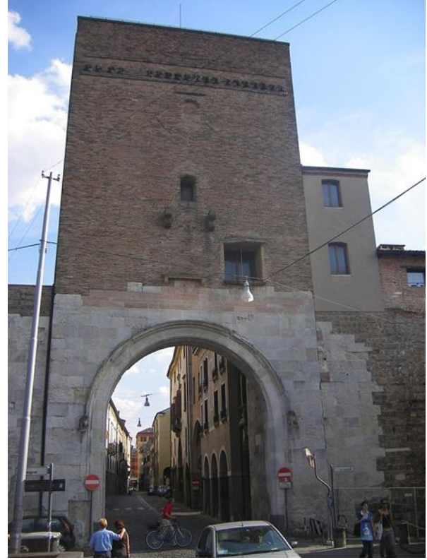
Figure 1. Ponte Molino Gate
