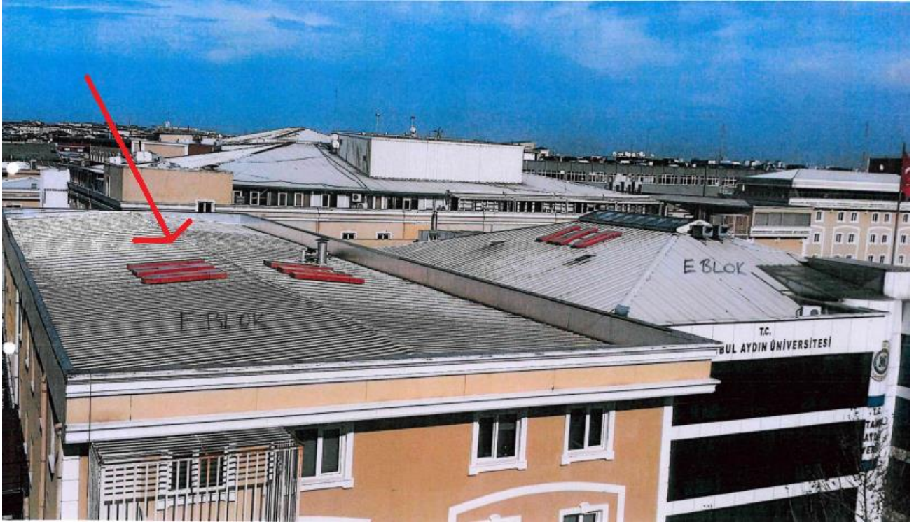
Figure 3. Rooftop of block F
