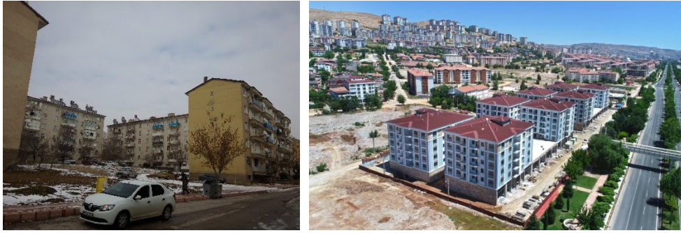
Figure 14: Abdullahpaşa neighborhood before and after the earthquake URL 4.
