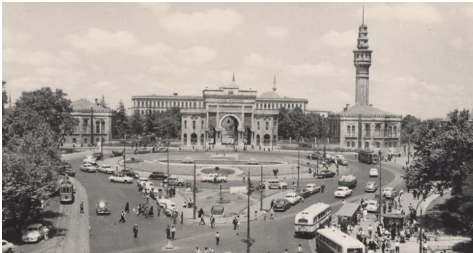
Figure 125. Entrance of automobiles to the square (INT-4)
