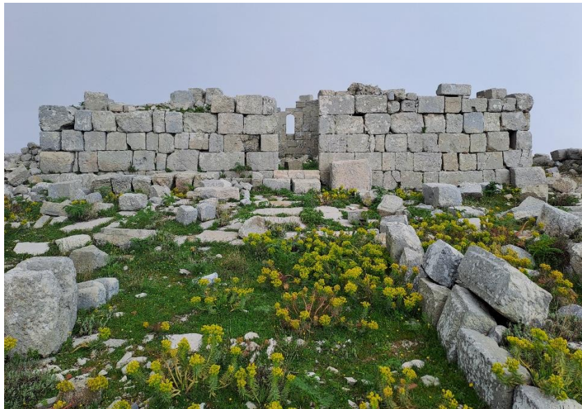
Figure 5: West exterior facade (M. Kaya, 2024)
