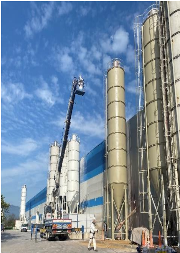
Figure 11. Second coat primer paint application of silos
