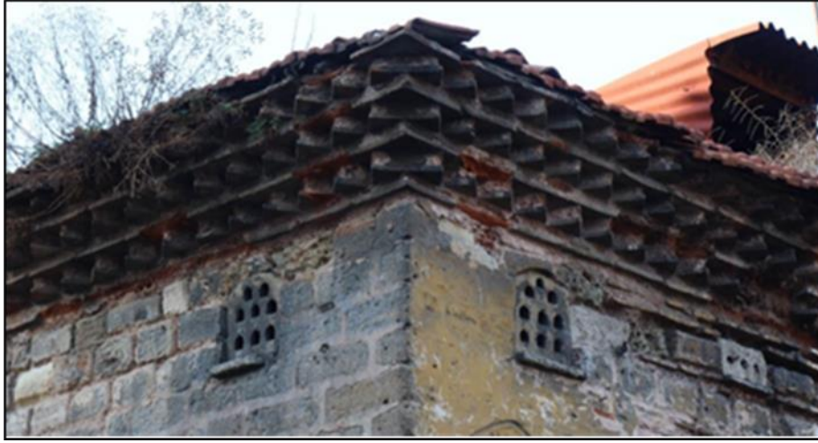
Figure 1. Image of the bird house in the outbuildings of the Tur-i Sina Church, İstanbul [11].
