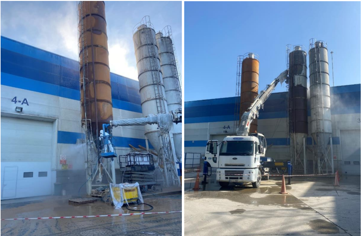
Figure 4. Wet blasting process
