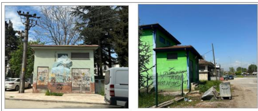
Figure 25. Appearances of transformer buildings located in the working area of Düzce/Uzun Mustafa neighborhood
