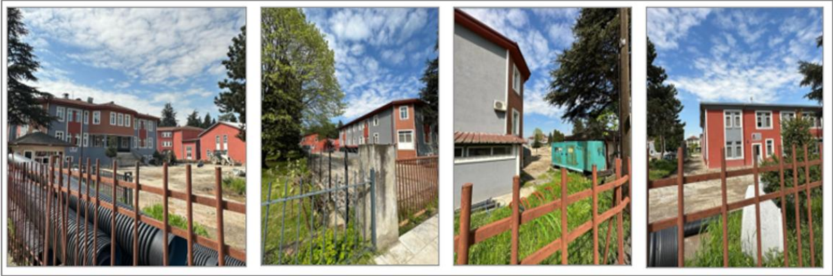
Figure 10. Views of Düzce Vocational High School and its surroundings located in the working area Düzce/Uzun Mustafa neighborhood
