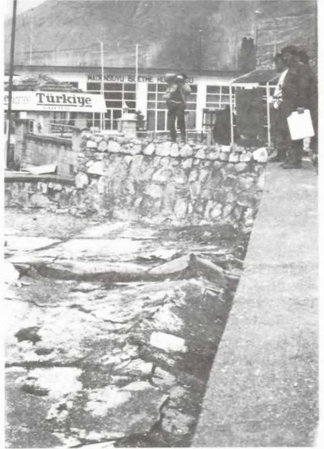
Figure 16 Compressional deformation structures developed at the heel of the area belonging to settling structure by the pool in the Ekşisu mineral water plant (photo from south to north).
