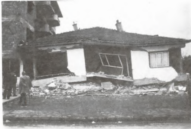
Figure 17 A totally non damaged building near the broken down three storey building in the city center. The only fissure in the multi storey building is the result of the strike of the next building (photo from west to east).
