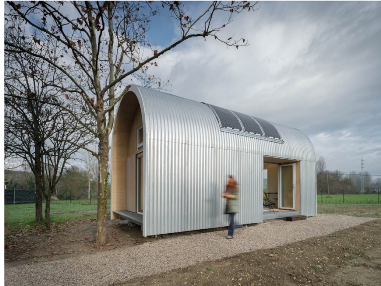
Resim 20. Mohma System Cabin, İspanya (Mohma System Cabin, 2024)
