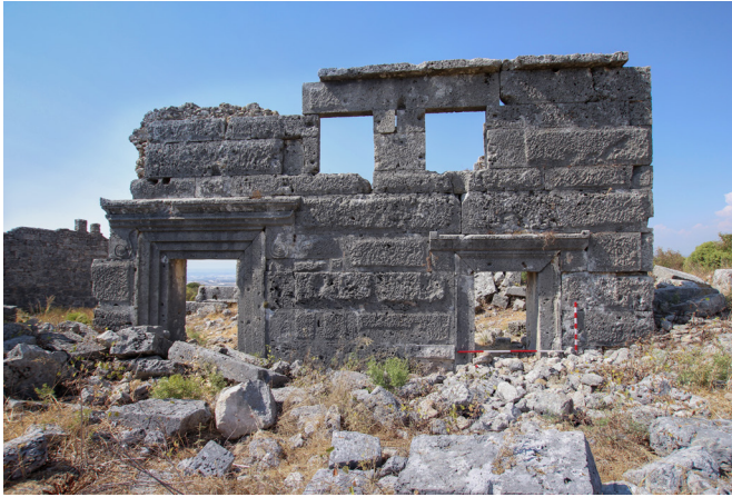
Fig.6 South facade of Andreion
