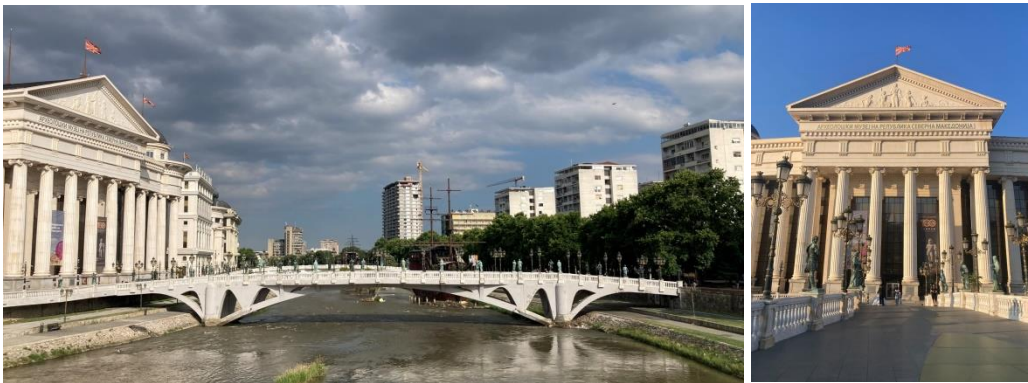
Figure 5. The Bridge of Civilizations (Oko Bridge)
