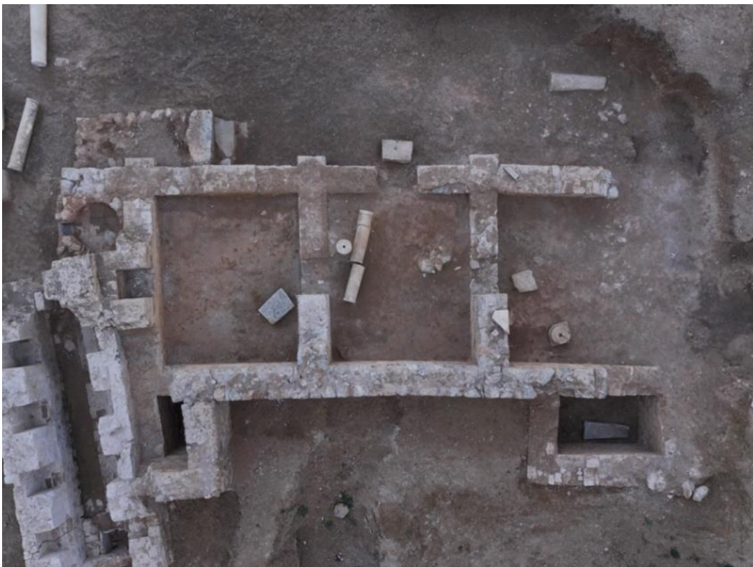
Figure 27: Aerial view of the workshop (IAM archive).
