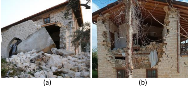
Figure 8. Poor quality, multi-leaves stone masonry buildings (a) Church of Mary, Samandağ, Hatay (Anadolu Ajansı, 2023), (b) English Protestant School, Samandağ, Hatay (Haber Global, 2023).
