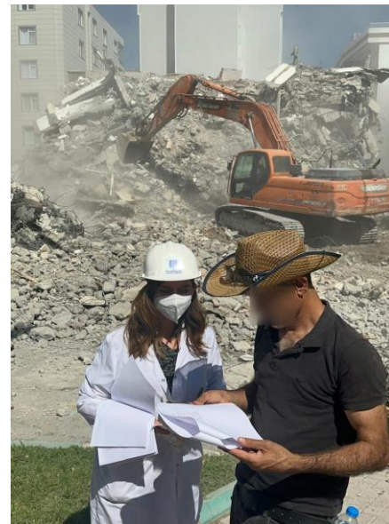
Figure 3. Survey of an individual from the SO group during the demolition
