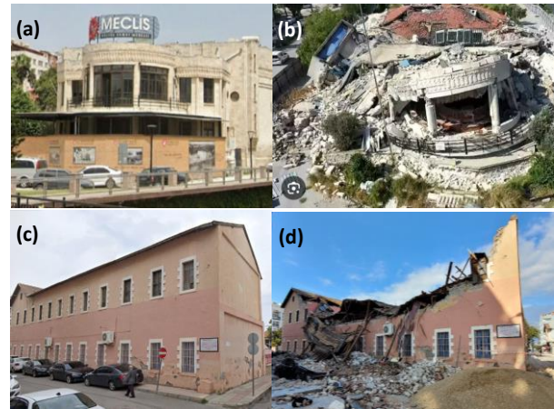
Figure 13. (a) Hatay Council Building before Kahramanmaraş earthquakes (Google Earth, 2022). (b) Hatay Council Building, damage after the earthquakes (CNN TURK, 2023). (c) Mithatpaşa Primary School, Kahramanmaraş earthquakes (Google Earth, 2022). (d) Mithatpaşa Primary School, damage after the earthquakes.
