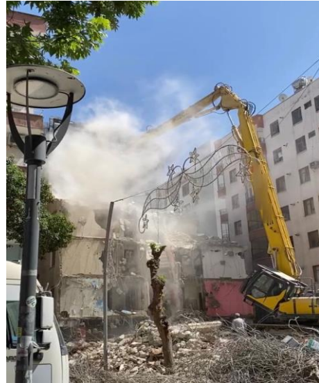
Figure 2. One of the demolition areas (Şanlıurfa)
