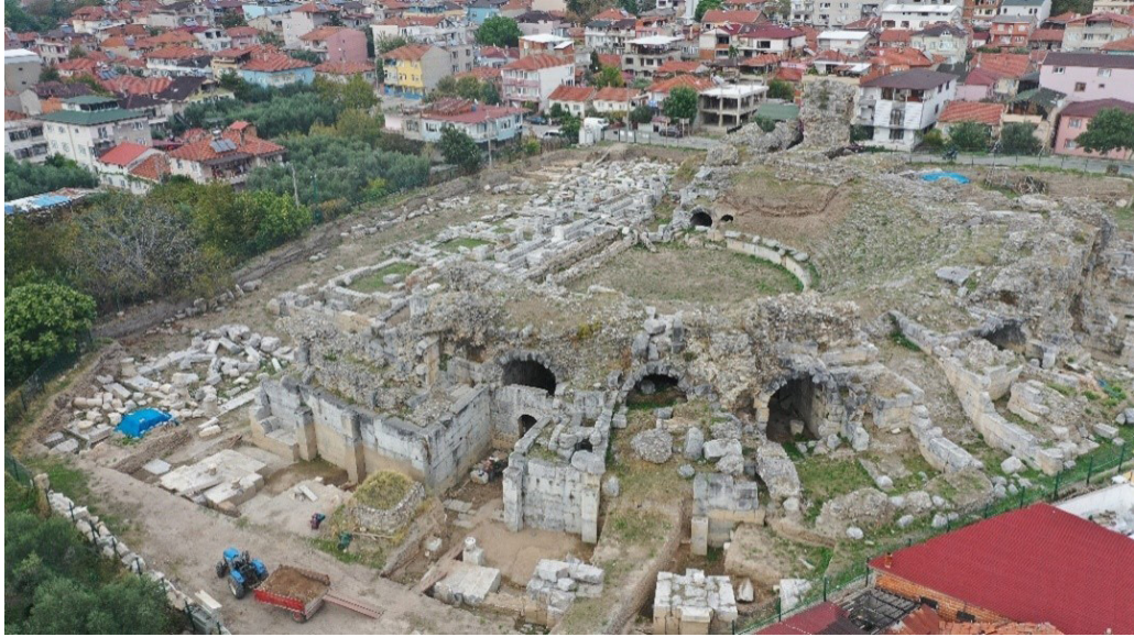
Fig. 7. Imposing vaulted infrastructure of cavea (courtesy of the Roman Theatre Excavation at Nicaea 2020)
