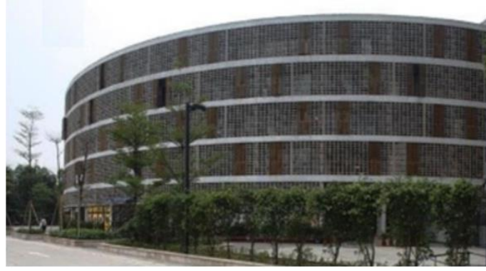
Figure 9. Façade with balconies (Aaberg-Jørgensen, 2011)
