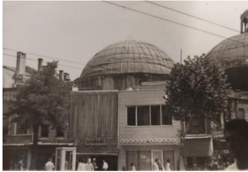
Figure 11. Reinforced concrete addition in front of the entrance of Çemberlitaş Hamam (1969) [28]
