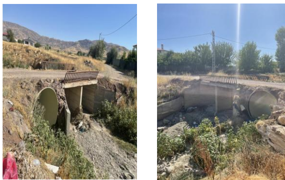
Figure 8. Culvert structure at the junction of Uluova and İkitepe streams.
