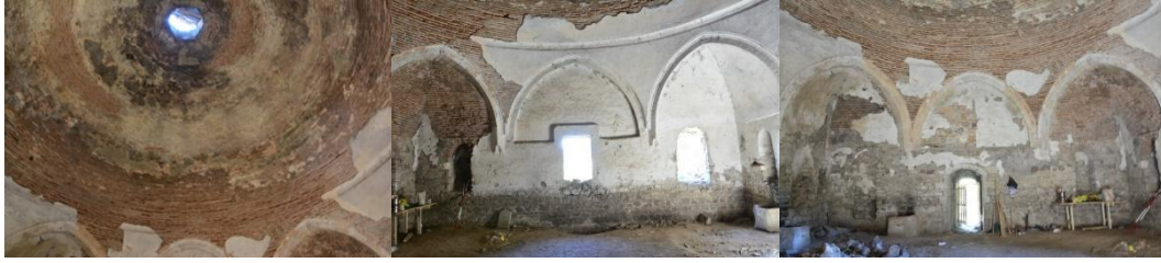
Figure 8. Interior view of the dome of the dressing room section, interior south wall of the dressing room section, interior west facade of the dressing room section
