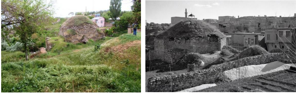
Figure 3. Northeastern facade views of the Hoca Hasan Bath in different periods Resource: (Archive photo MVGM, 2025)
